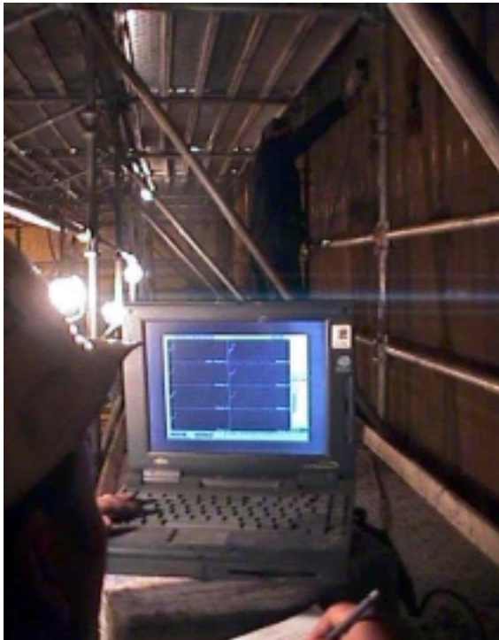
Testing being performed on waterwall tubing inside an actual boiler.
