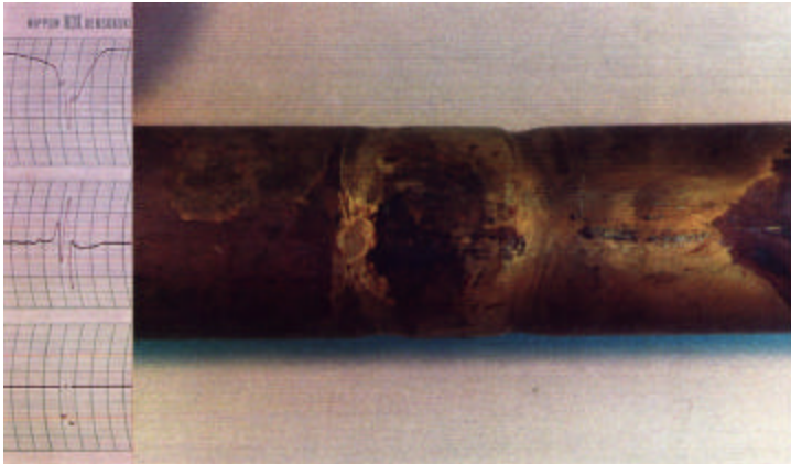
Ammonia attack at the tube support
