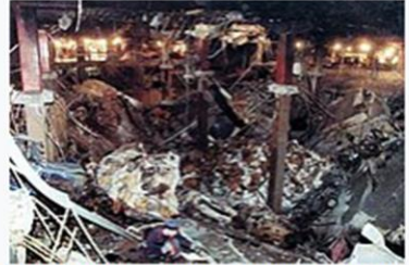
Underground damage after the bombing
