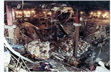
Underground damage after the bombing
