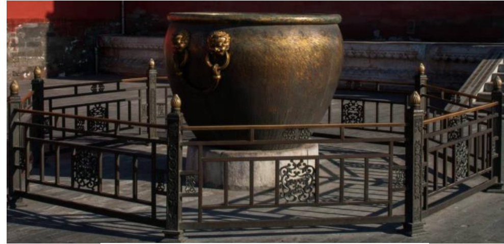
Fire suppression system
